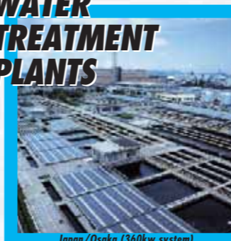
Japan/Osaka (360kw system)
