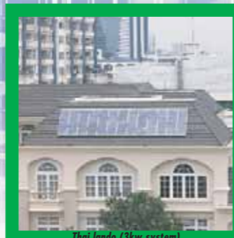
Thailand (3kw system)
